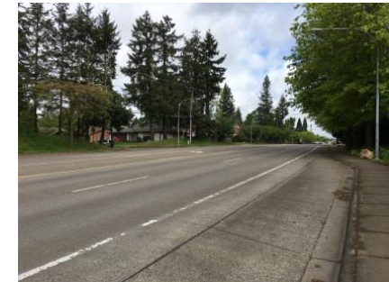
Facing north from SW Jay Street
